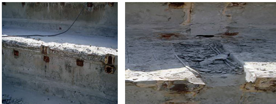
Fig. 1. Reinforced concrete construction damages of folding panels after cutting off encrustation from concrete repair mortars
