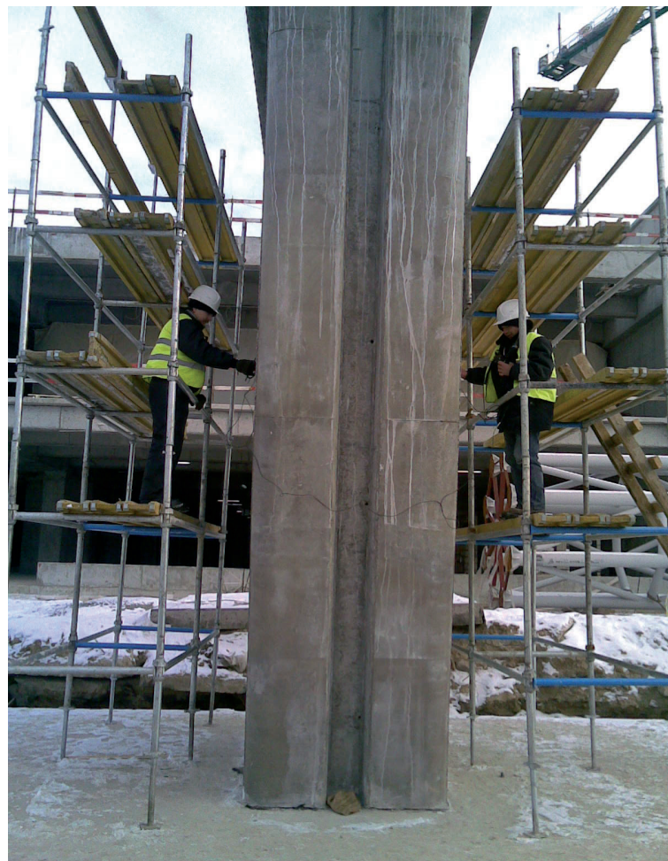
Fig. 1. Ultrasonic testing to determine the concrete strength in monolithic structure.
