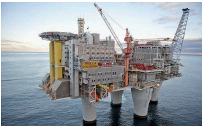
Fig. 6. Ice-resistant stationary gas production platform Troll-A in the North Sea, installed at 300 meters depth of water (Norway)
