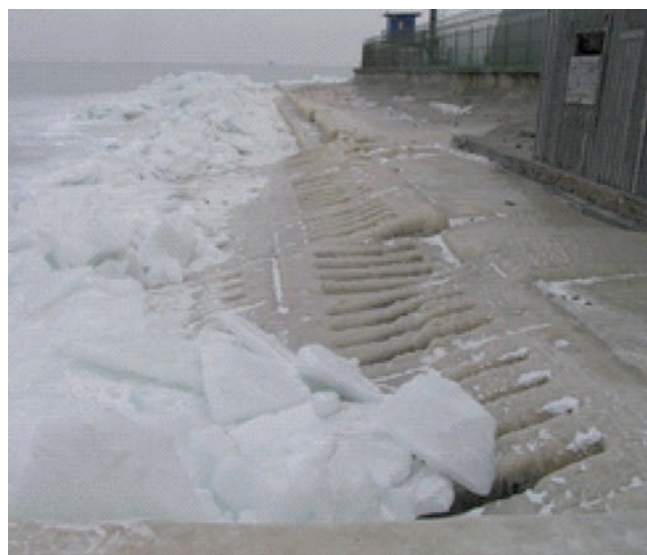
Fig. 3. The hummocking of an even ice field on the shore protective structure of the sloping type (PJSC Odeskabel)
