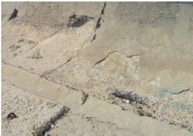
Fig. 5. Wave-breaking wall of the shore protection structure (PJSC Odeskabel)
