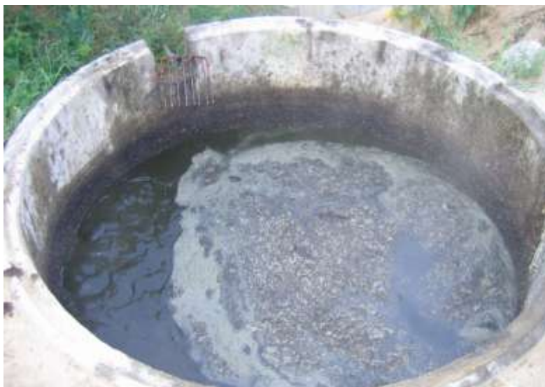
Fig. 4. Preliminary storehouse for liquid fats used for feeding the anaerobic fermentation chamber (photo: Jan Cebula)
