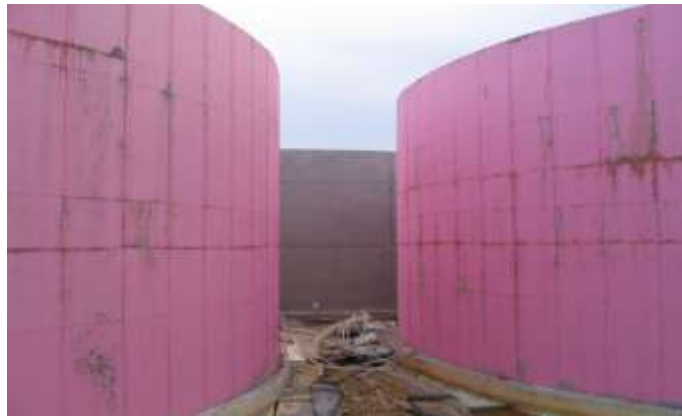
Fig. 6. Fermenters made of reinforced concrete and insulated with polystyrene foam (photo J. Cebula)
