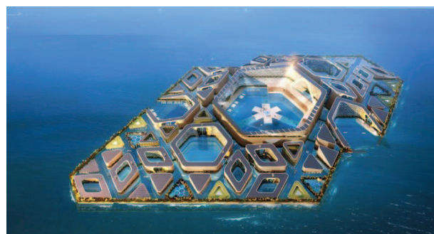
Fig.3. City Water Project, China Communications Construction Company (CCCC-FHDI) & AT Design Office, China, 2014
