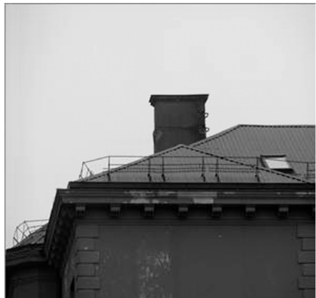
Fig. 8. LatPos antenna installation location (Valka gymnasium)
