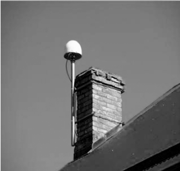
Fig. 9. Base station Palsmane attachment to the chimney
