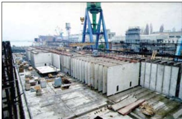
Fig. 1. Formation of the steel-concrete pontoon of the floating dock with the buoyant power of 25,000 t in the docking chamber of the plant
