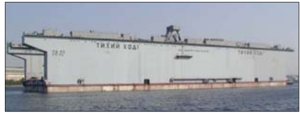
Fig. 6. Repair composite floating dock with the buoyant power of 13,500 tones before delivery to the Russian Federation
