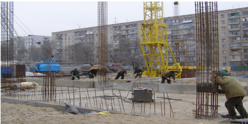
Fig.5. The loading of a flat precast cast-in-situ deck during the test
