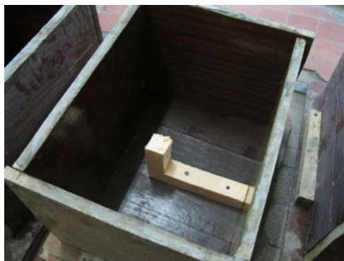
Pic.1. The formwork form with the liner made from form polystyrene.
