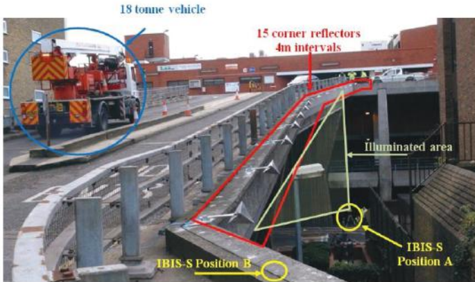
Figure 7. The lorry passing over the bridge, with data acquisition at position A
