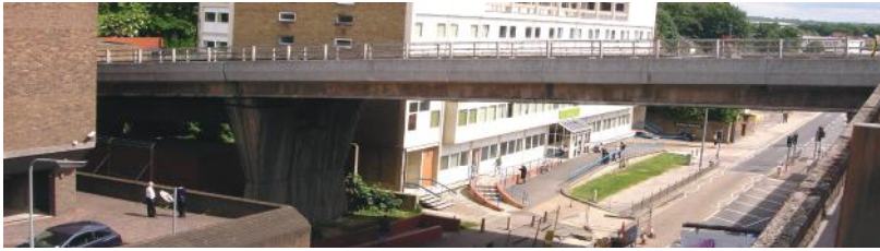
Figure 1. General view of the Pentagon Road Bridge
