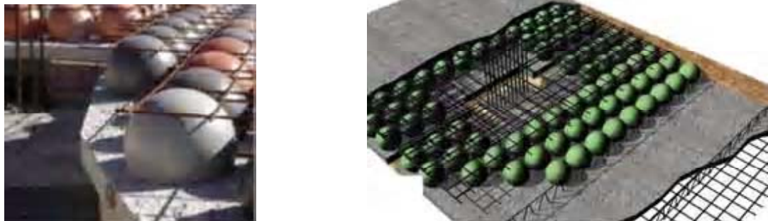
Figure 6. Flat slabs with ball-shaped inserts – Bubble Deck.
