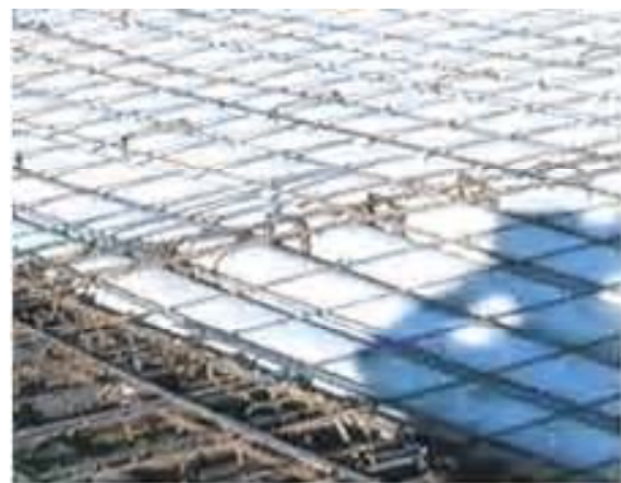
Figure 7. Solid slab installation with pipe-shaped voids.
