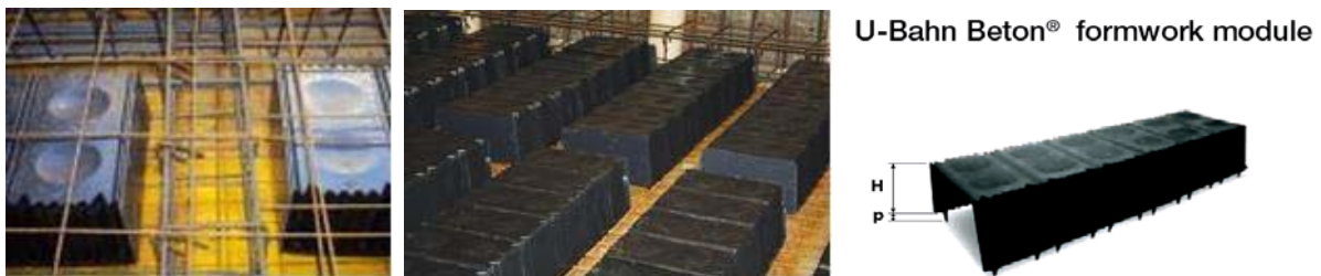
Figure 2. Installation of a solid slab using the U-Bahn beton system.
