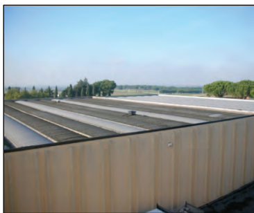
Fig.1. Roof in asbestos
