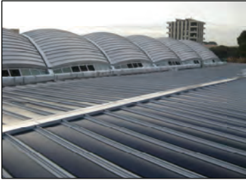
“Eutecna Energia” different realizations in corporation with “Elleemme” Fig.8. BIPV in Roma – kWp 31,00
