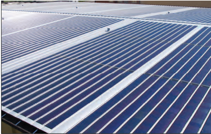
Fig.7. Realization of BIPV, thermal insulation and active ventilation
