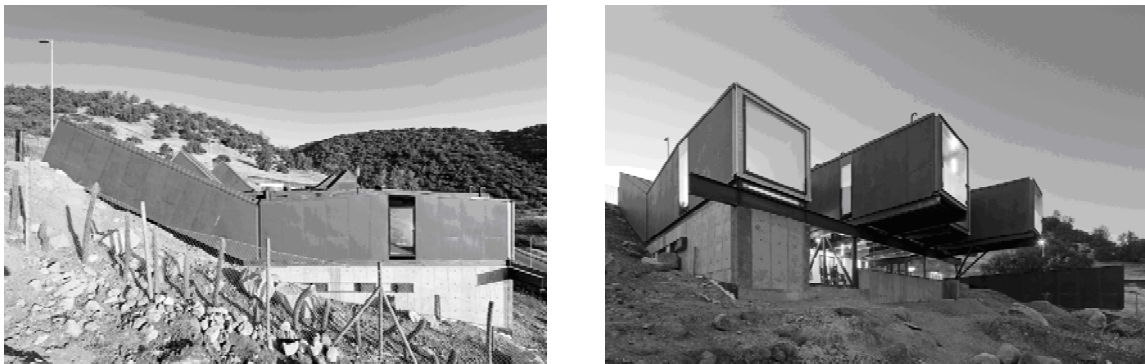
Picture 2 – Container house in Santiago, Chile.
