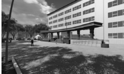
Picture 4 – The appearance of educational building.
