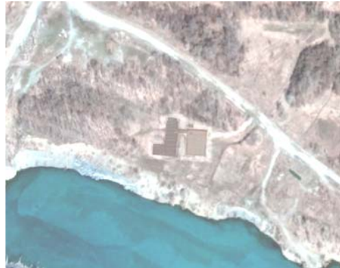
Fig. 4. General view of a building under construction and a portion of the modeled area near the slope
