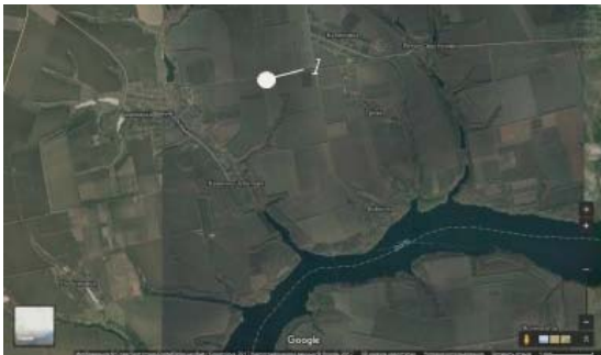
Fig. 1. GOOGLE's image of Ammonia Pump Station: l – pump station
