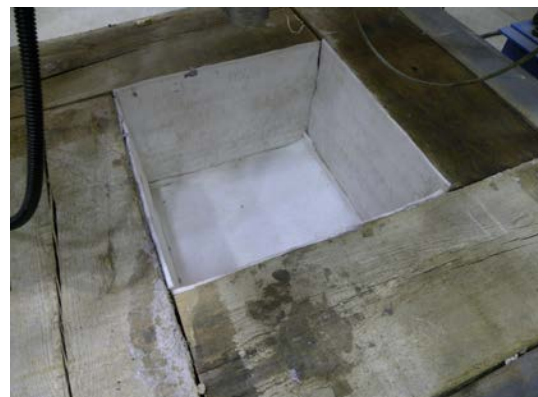
Fig. 2. The «box» built from wooden sleepers
