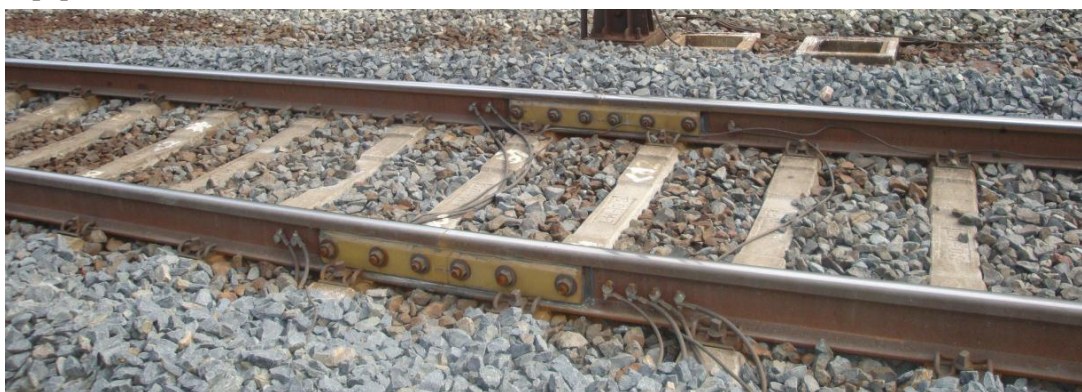
Fig. 1. Glued insulated rail joints with special fibre-glass reinforced plastic (polymer-composite) fishplates (brand: APATECH) in railway track (authors' photo)
