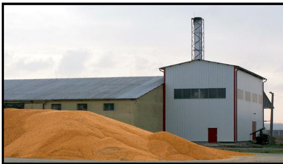
Picture 4 The broiler after reconstruction view
